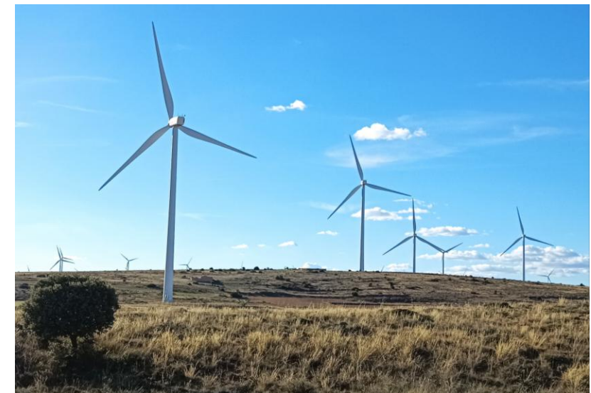
Onshore wind energy
